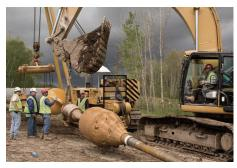
For large rivers or certain sensitive crossings, directional drilling is an appropriate and preferred construction method, depending on geologic conditions and other factors. HDD construction is considered suitable for large river crossings, extreme congestion (e.g. crossing rail yards), or other unique site-specific situations because it minimizes impacts on the area above the drill.
